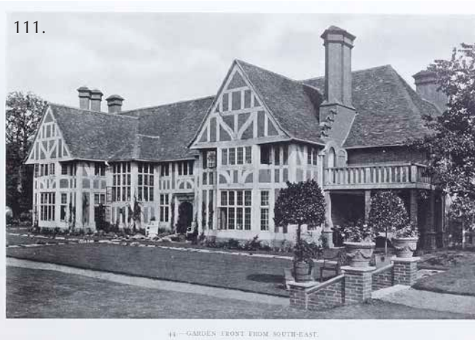
44 - GARDENS - FRONT FROM SOUTH-EAST.
